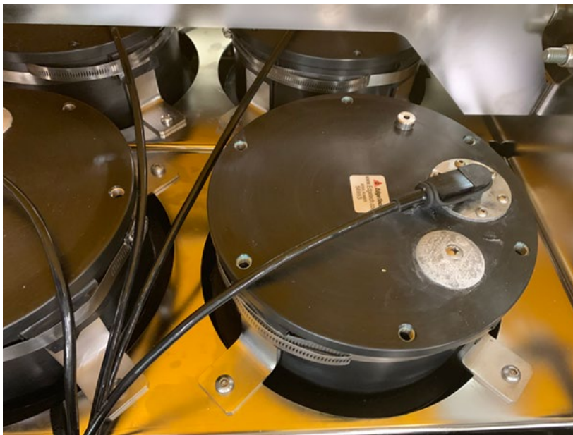
Figure 6-10: Correctly Installed Sub-Bottom Transducer
